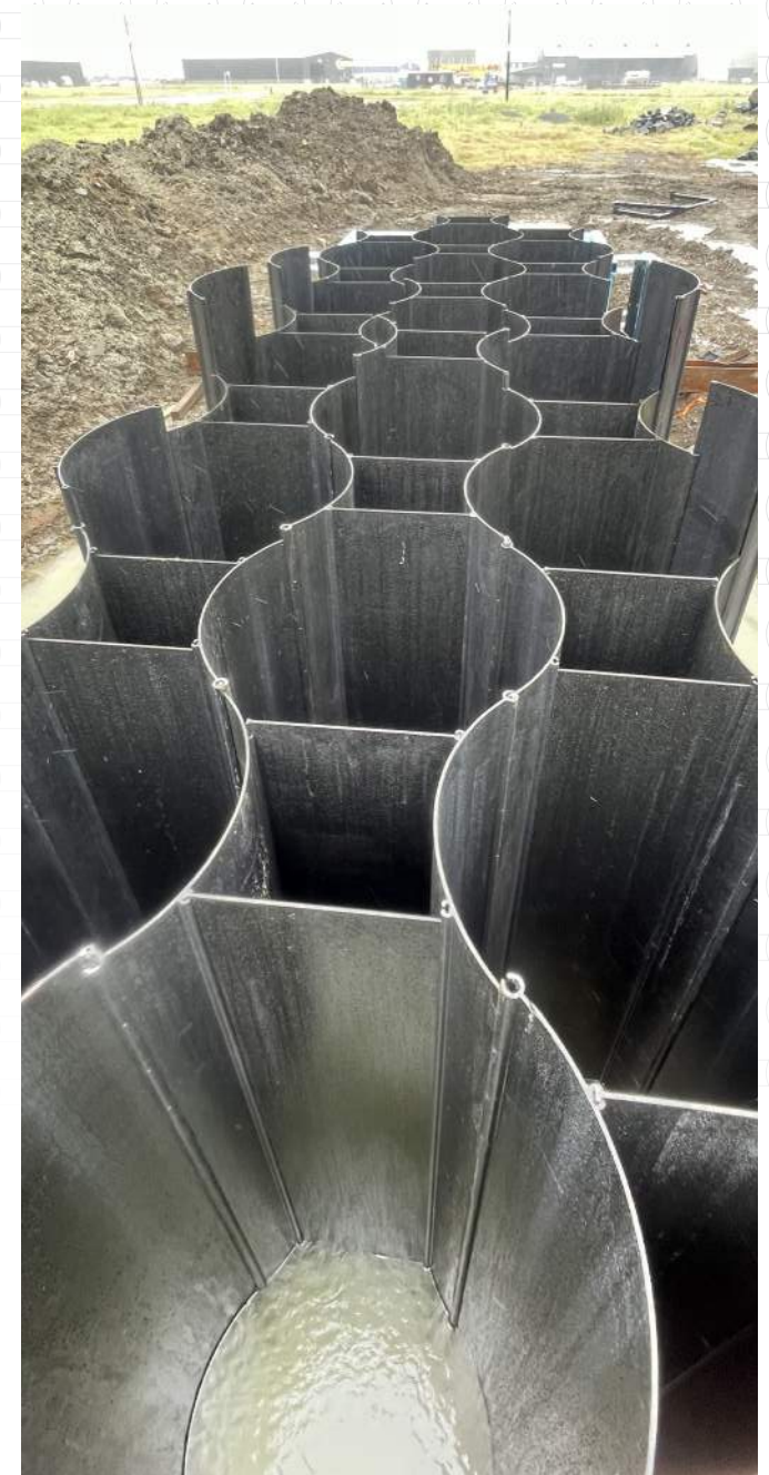
CombiLoc™ Trial Installation
